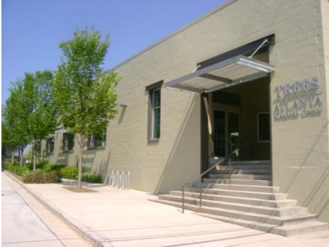
Front Exterior of Kendeda Center
