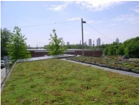
Rooftop Garden and Solar Panels
